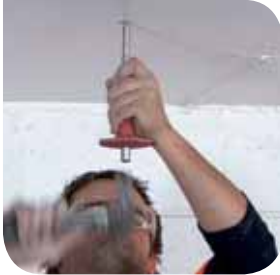
1. Measure off and fit bulldog fastenings.
