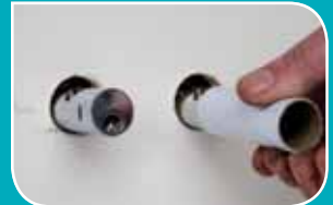
When ready to fit appliance / fixture remove protective cardboard cover and slide over flange.
