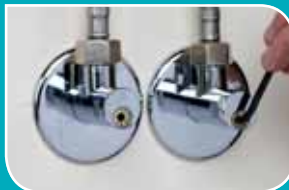
Install Iso-Filter and/or Iso-Adaptor if required.
