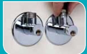
Firmly hand tighten the IsoNipple and secure the O-ring seal with a spanner.
