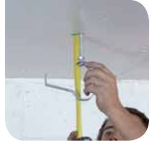
3. Measure fall and spin on top nut approx 5mm above the measure.
