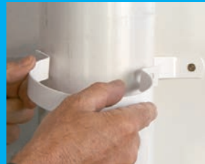
Step 3 – Place pipe into bracket base.
